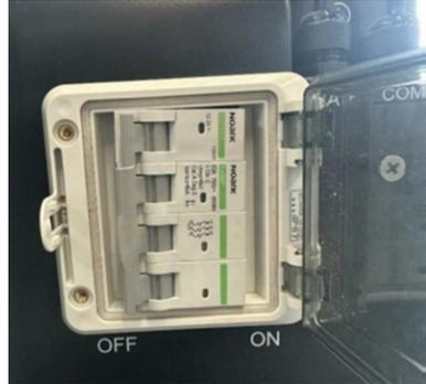
2. Switch on the DC switches on all battery modules and switch them off again after approx. 6-9 seconds. Perform this process a total of three times on each battery module.
